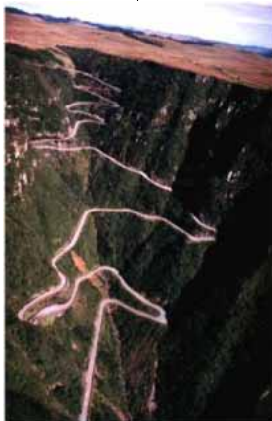
Figure 19 - SC-438 road from Lauro Muller to- São Joaquim and the top of the Serra do Rio do Rasto.
