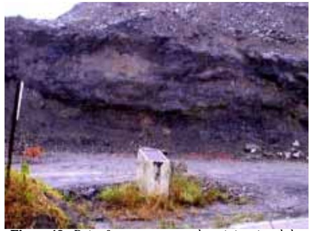
Figure 12 - Point 9 concrete post where it is printed the outcrop description.
