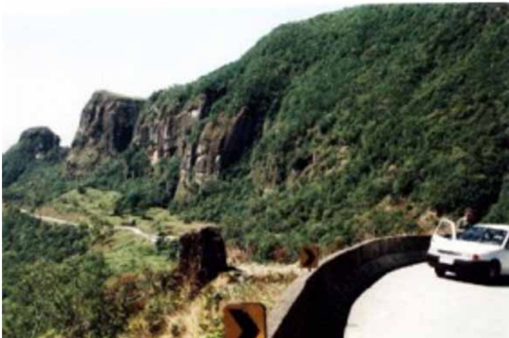
Figura 13 - Section of the road by the 14 and 15 points (photo by Wilson Wildner).
